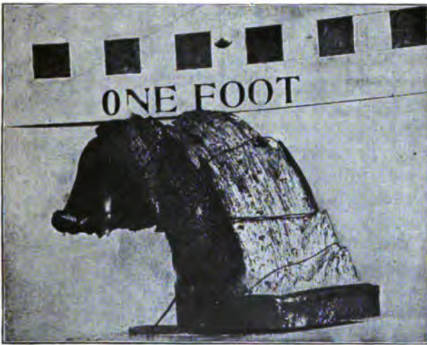
Fig. 75. Barked Wrought Iron, Stumm.
